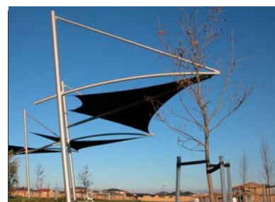
Shade Structure by Oasis
